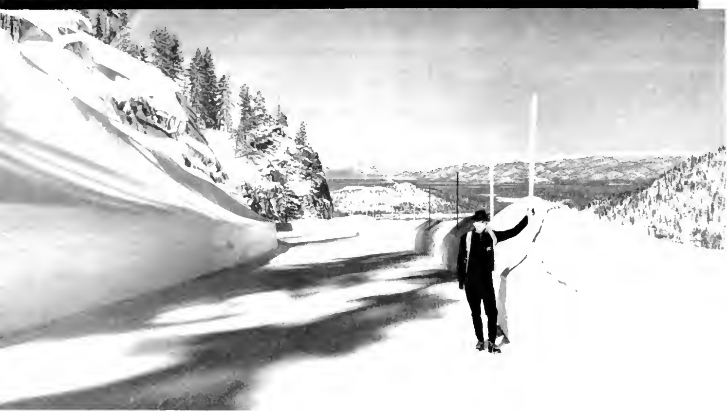
Scene on Echo Summit after snow removal operations. Depth of snow pack is clearly shown in this picture
